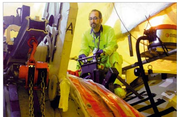
Fig. 2. Removal of contaminated layer from the metallic assembly [17]
